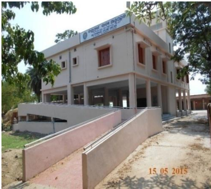
Balarampur MCS in Basudevpur Block under NCRMP, World Bank funded
